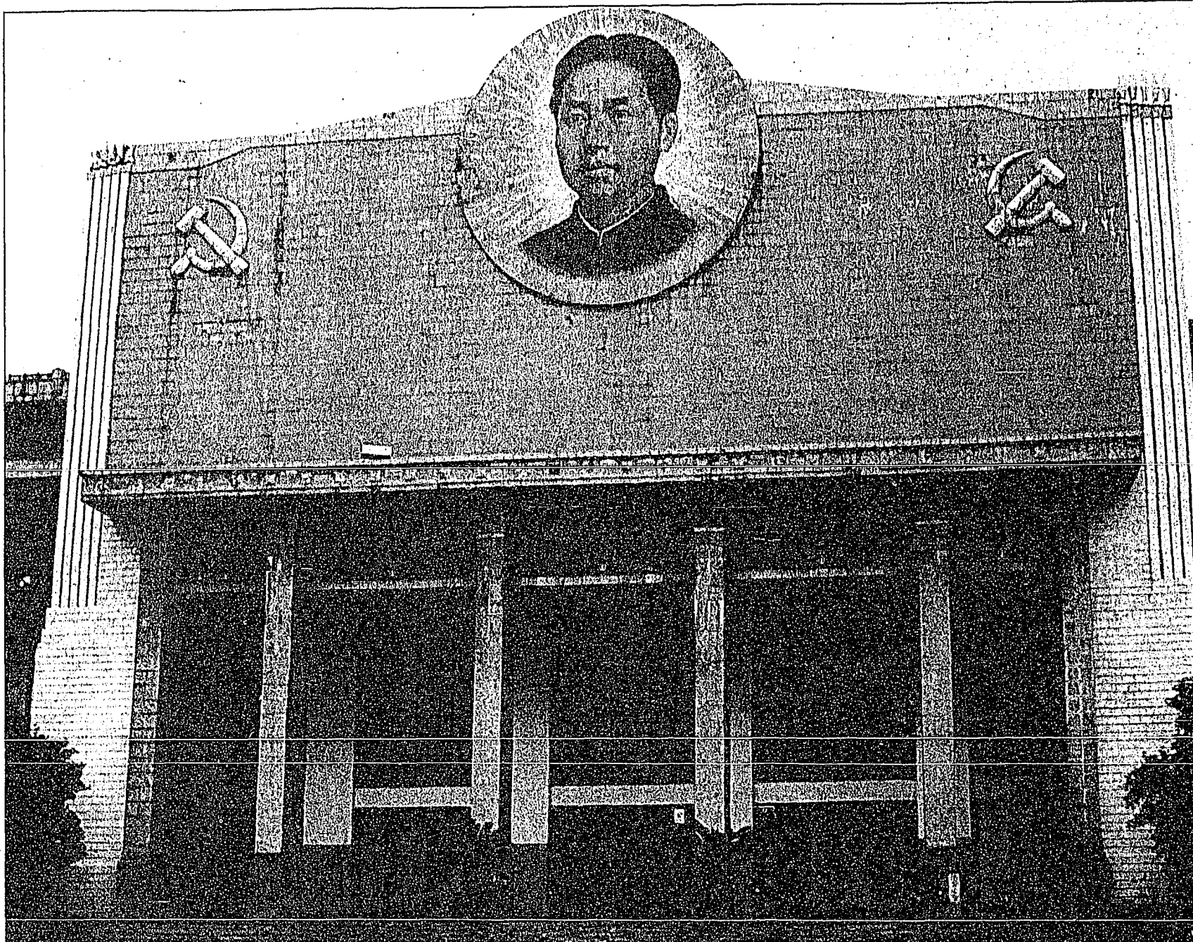
● Fallen idol . . . the Mao Zedong Memorial Hall is cracked and neglected, but work is under way to get it back into shape in time for the centenary celebrations.
